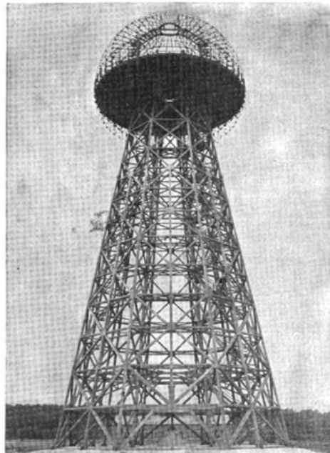
FIG. 2.—TESLA CENTRAL POWER PLANT AND TRANSMITTING TOWER FOR WORLD TELEGRAPHY, AT WARDENCLYFFE, LONG ISLAND, N. Y.
